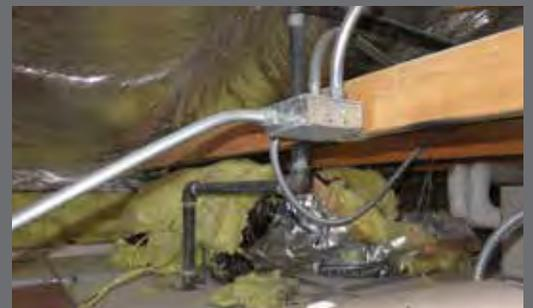
Foil-faced air permeable fiberglass insulation that had been installed under the roof deck was removed and replaced with ccSPF insulation.
