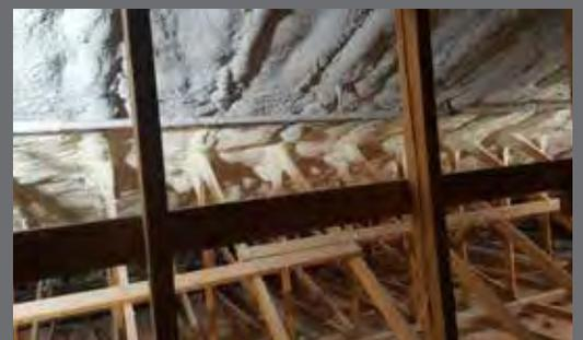
CcSPF effectively sealed the complex roof structure providing the required air tightness.
