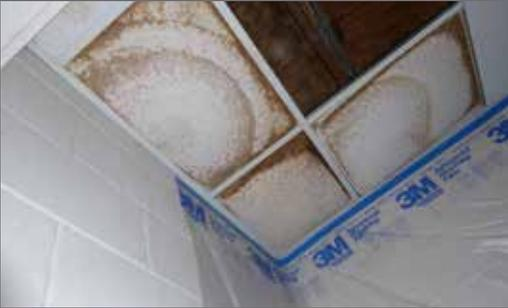
Prior to ccSPF being installed, ceiling tiles within the school were frequently damaged due to moisture issues and had to be replaced.
