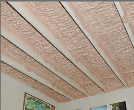
The new wall system sprayed flawlessly, adhered well and had a smooth finish.
