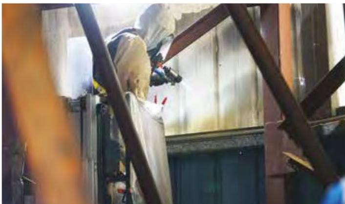
The ccSPF application was challenging due to the silo's 28 ft. height and the many obstructions that had to be avoided while spraying from a lift.
