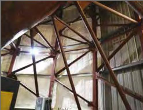
Adhesion to the metal silo wall was important, as well as the foam's ability to provide an air and moisture barrier.
