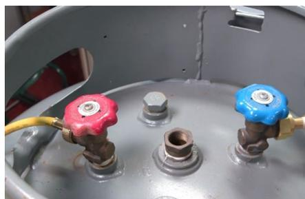
5. If both these requirements are met, connect the liquid discharge line and secure tightly.
