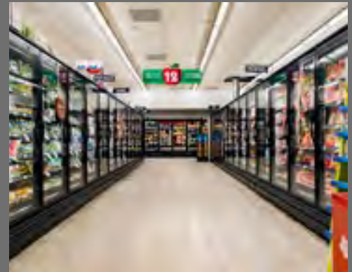
The Zero Zone closed-door display cases enhanced food presentation while improving energy efficiency.
